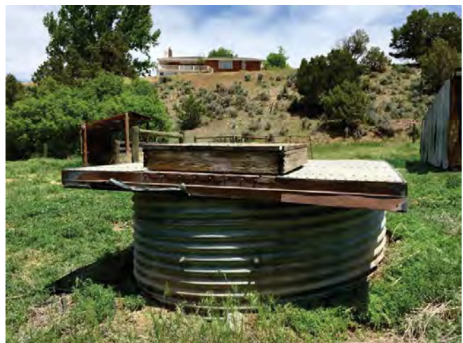
Looking north at domestic spring manhole in the Bull Pen parcel (6/6/16).
