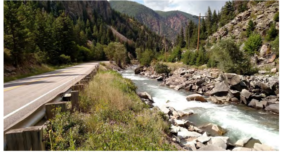
Alternative A: Looking north
