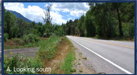
A. Looking south - Vegetated Area
