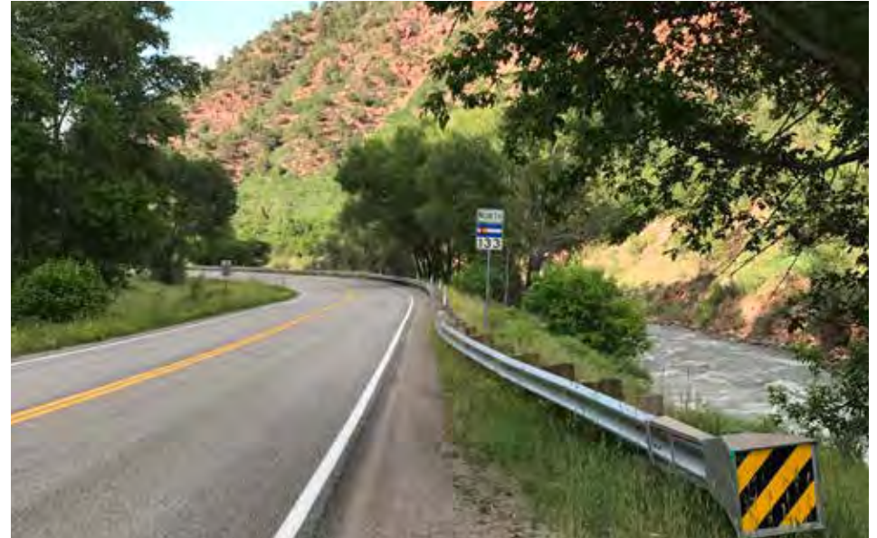
Alternative A: Looking north along the highway
