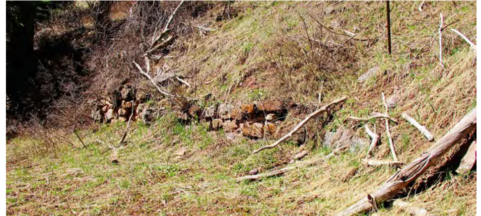
Remnants of the Rock Creek County Road can be found throughout the valley, including the original platform, old bridge abutments and hand-built retaining walls like the one pictured here, at the Drool Open Space.
