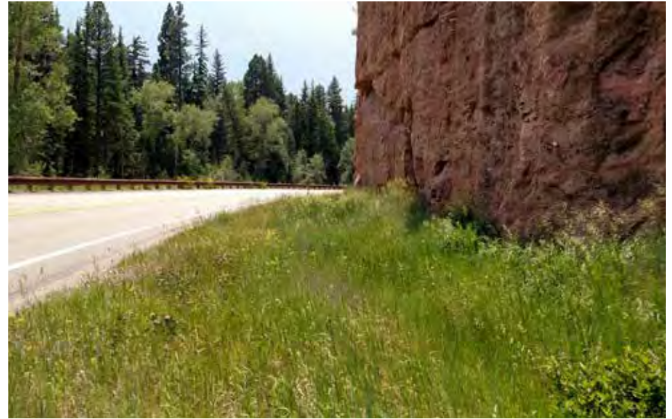
Alternative A: Looking south along the highway where a trail would hug the vertical rock wall
