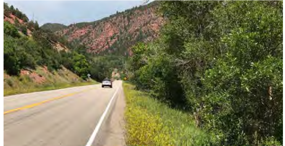
Alternative A: Looking North
