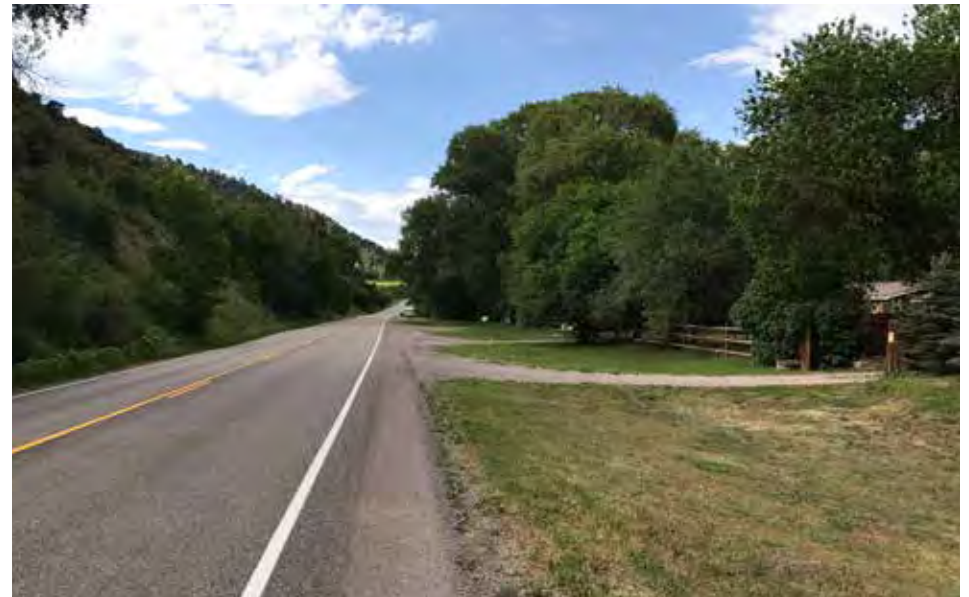
Alternative A: Looking north along the highway where the trail would cross a number of driveways
