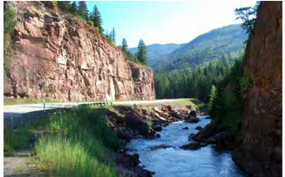
Alternative A: Looking north along the highway
