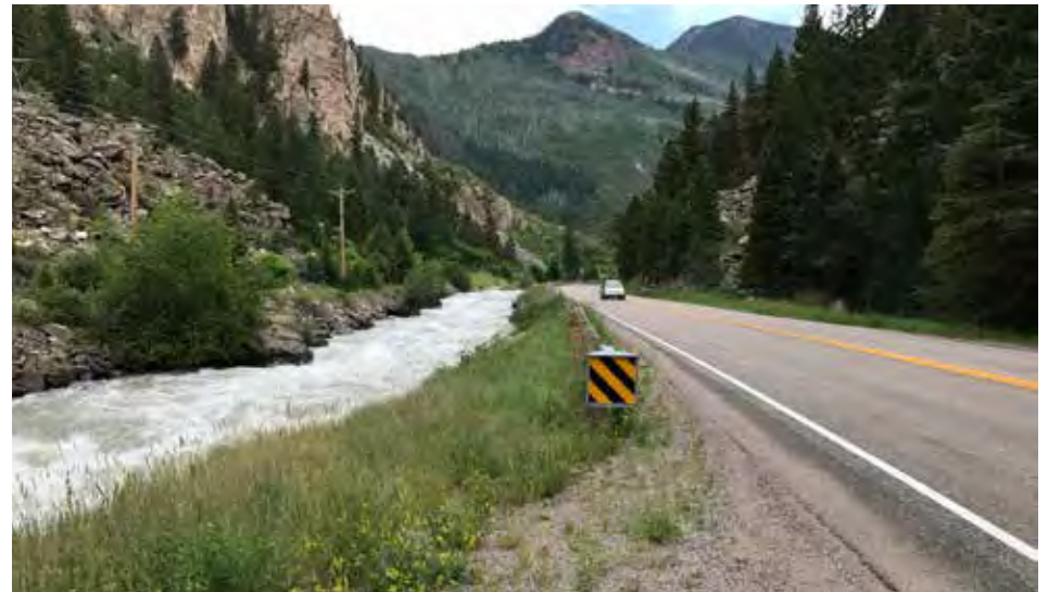
Alternative A: Looking south along the river
