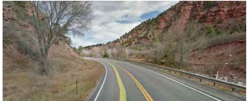
Alternative A: Looking North
