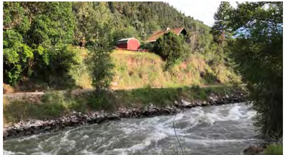
Alternative B: Looking toward the road platform on the east side of the river
