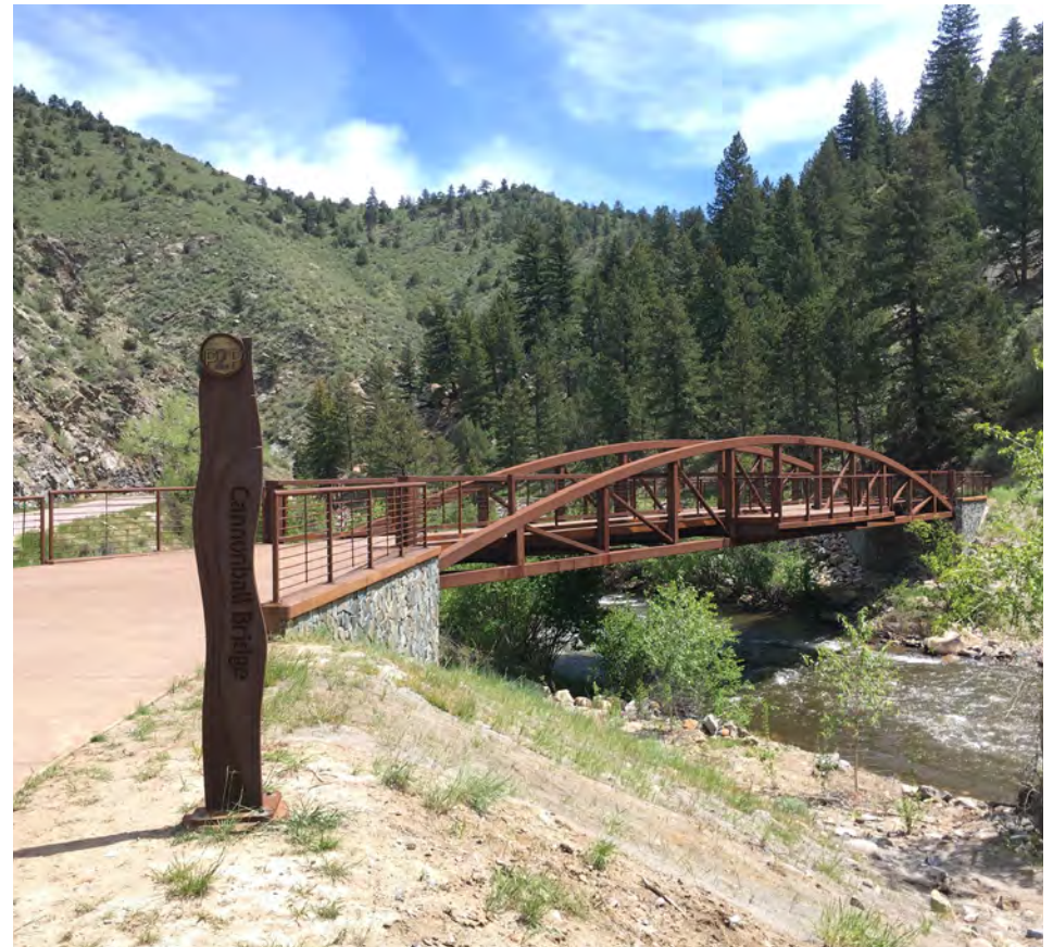
Example of a bridge representing Typical Section 7A, from the Peaks to Plains Trail in Jefferson, County, CO.
