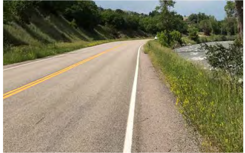
Alternative A: Looking north along the highway
