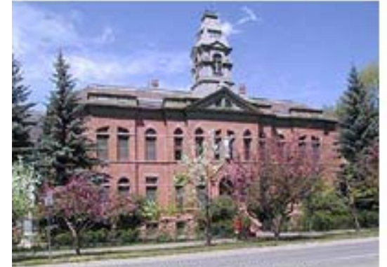
PITKIN COUNTY COURTHOUSE
