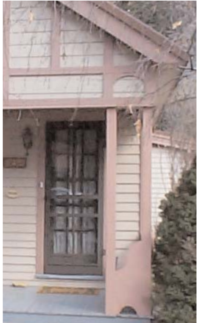
a detail from a house on the Boulevard
