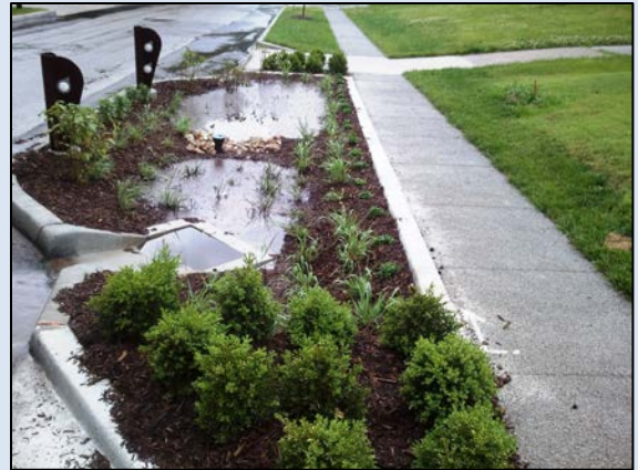
Figure 20: This rain garden in Kansas City's Marlborough neighborhood was built as part of the improvements in the Middle Blue River Basin.
