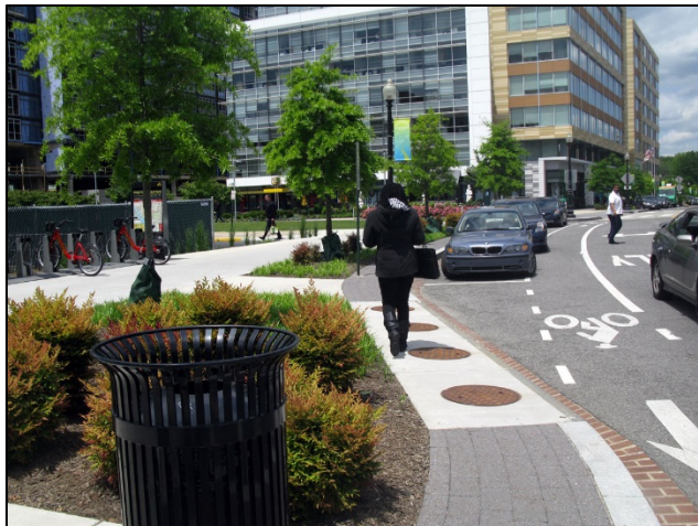
Figure 16: Fourth Street SW in Washington, D.C., is a green and complete street, with a bike lane, a wide sidewalk, and planting areas.
