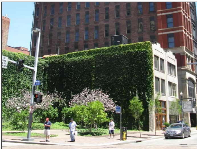
Figure 28: Green walls, such as this one in downtown Pittsburgh, Pennsylvania, can help reduce the heat island effect.
