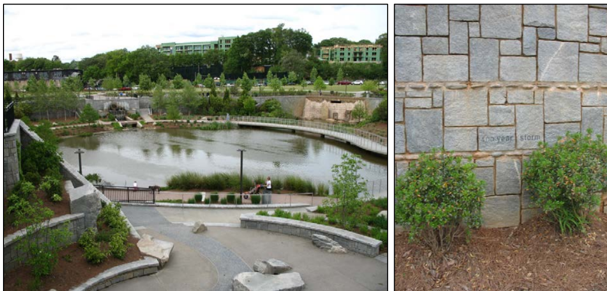
Figure 5: Atlanta's Historic Fourth Ward Park (left) was designed to capture excess rainfall and reduce downstream flooding. It saved the city $15 million in infrastructure costs compared to a conventional stormwater facility. Lines on the park's walls mark the 100-year and 500-year flood heights to help educate residents (right). The park is a beautiful amenity for the neighborhood, spurring new development nearby. 25
