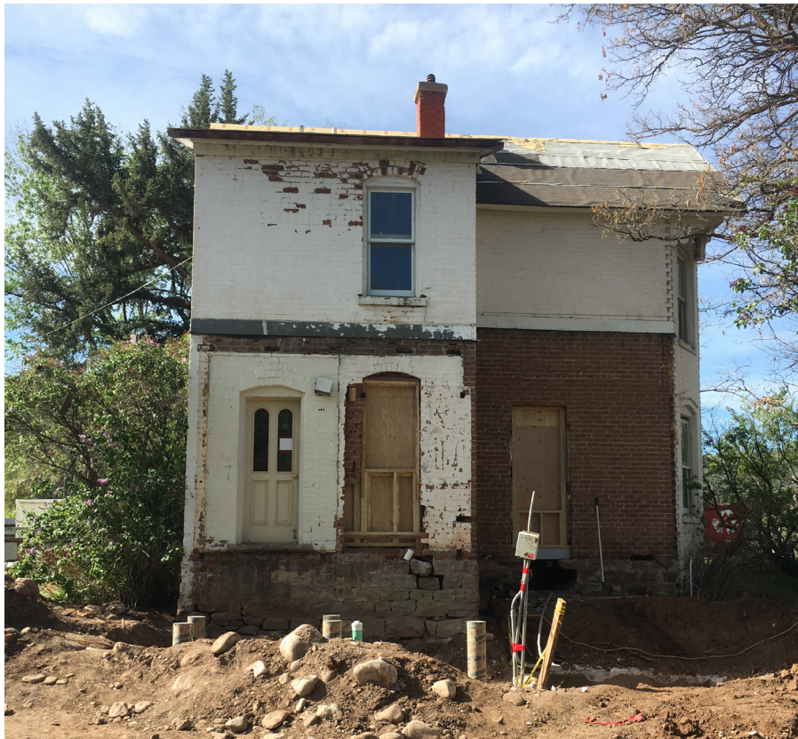
The rear of the house today, with a new back porch (above) and the house in mid-construction (below), after two non-historic, rear additions had been removed.
