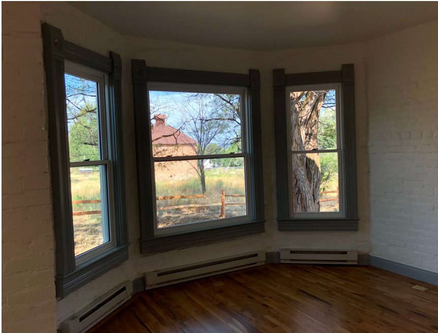
The view from the dining room, and stairway to the second floor.
