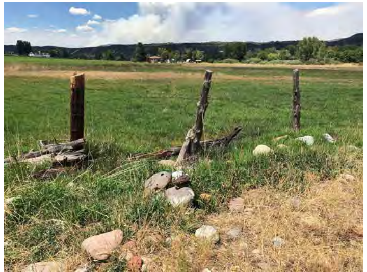
Fences in various states of disrepair across the property will be repaired or removed.
