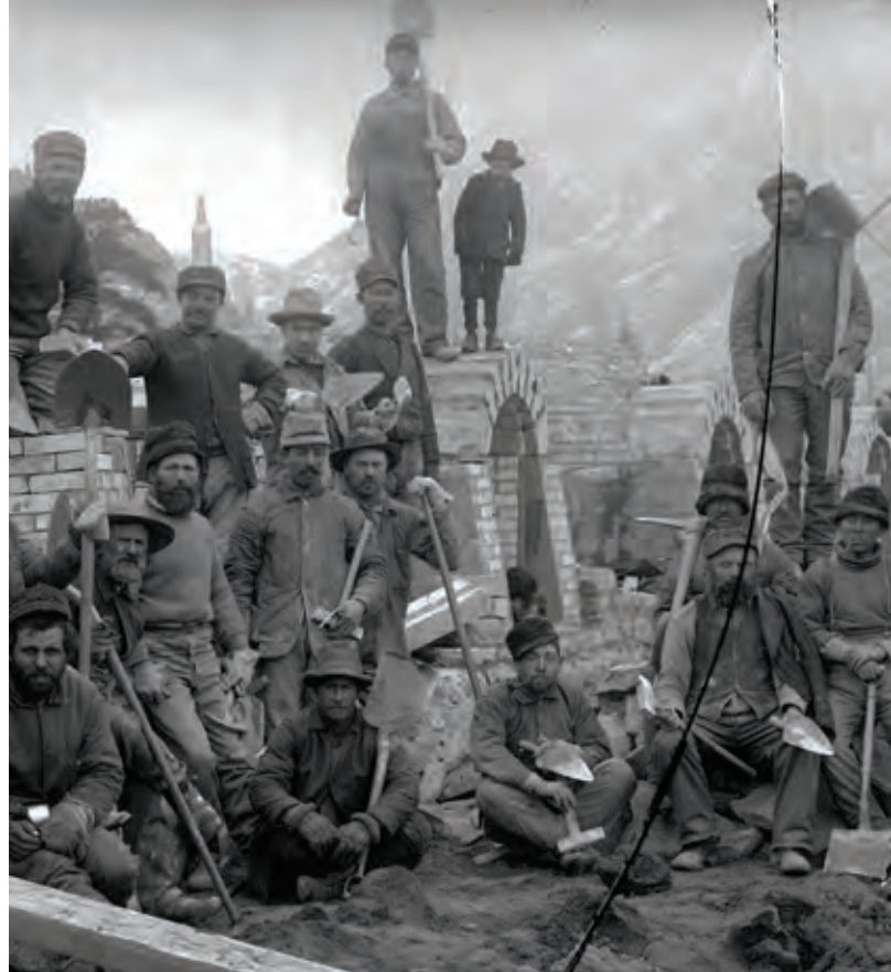
Workers pose for a photo during construction of the Redstone coke ovens in 1902. Photo source: Aspen Historical Society, Masterson Estate Collection
