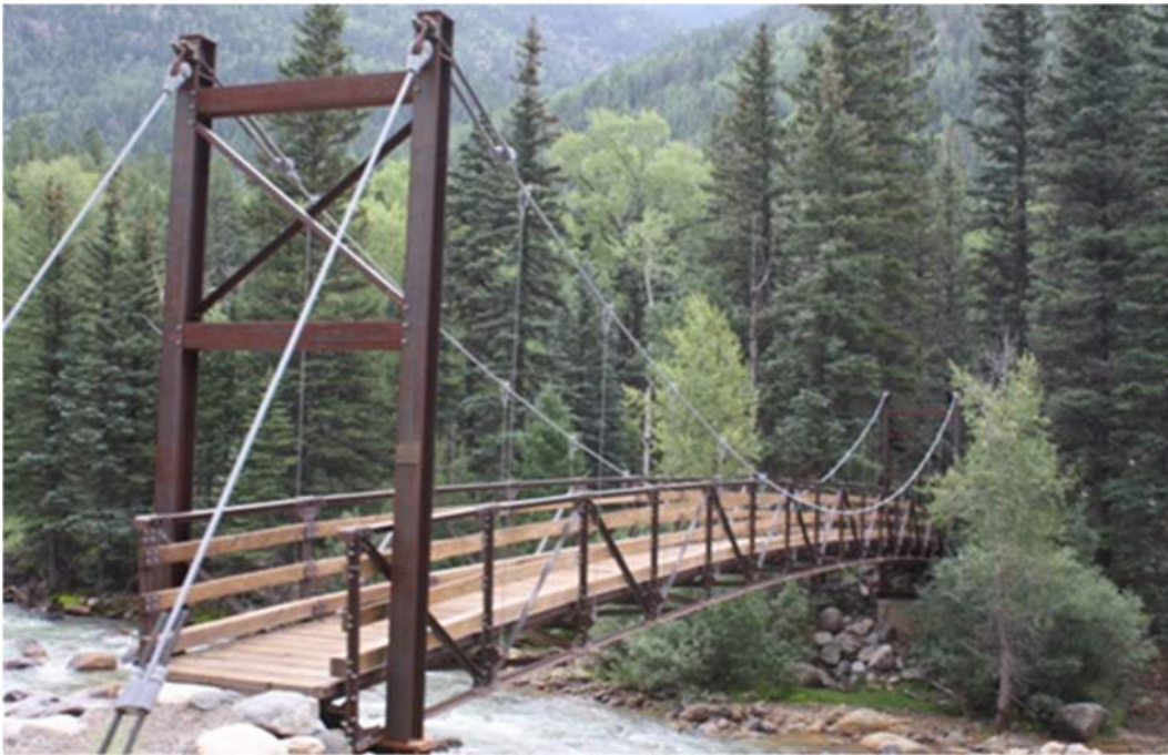
Figure 15: Elevation view of the suspension bridge at the Needleton Trailhead, San Juan National Forest, CO
