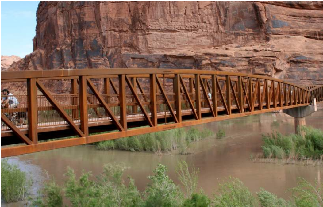
Figure 9: Colorado Riverway Bridge in Moab, Utah. Multi-span prefabricated weathering steel pony truss (courtesy of Contech Engineered Solutions)
