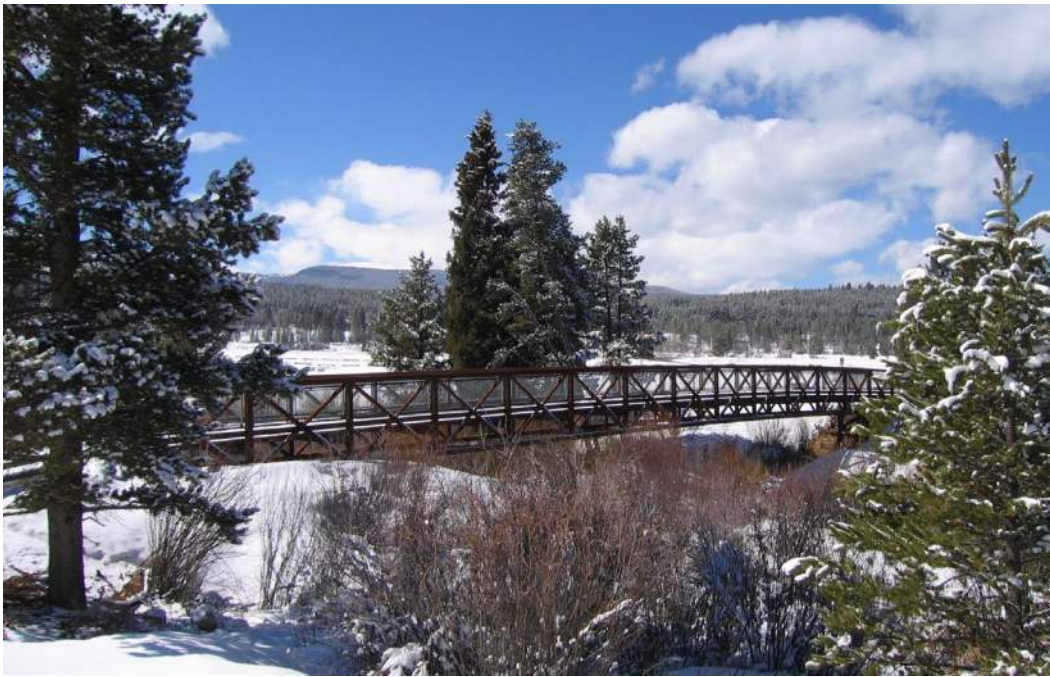
Figure 8: Rendezvous Development Bridge over the Fraser River in Winter Park, Colorado (courtesy of Big R Bridge)
