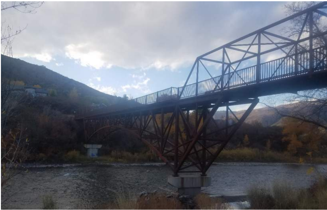
Figure 10: 14 th Street Pedestrian Bridge in Glenwood Springs, Colorado. This is a more custom option with a main span deck truss and through trusses in the approach spans.
