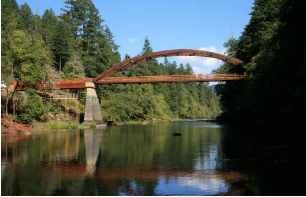
Figure 14: Tioga Bridge over the North Umpqua River in Oregon. Tied arch bridge with concrete piers (courtesy of Western Wood Structures)
