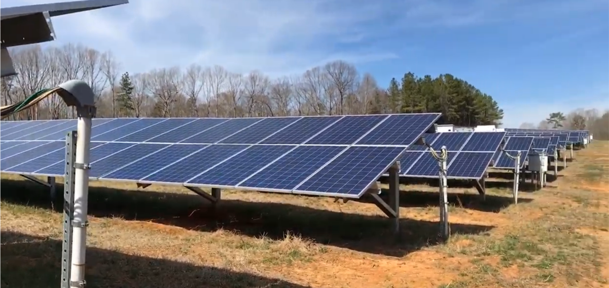
Figure 2. Sample Fixed Tilt Solar Array
