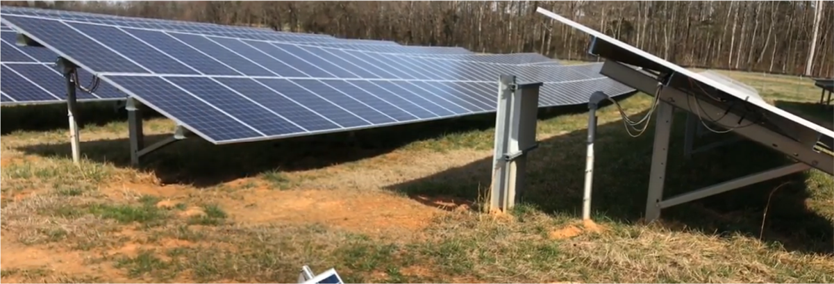
Figure 3. Sample Fixed Tilt Solar Array
