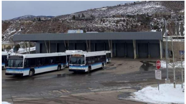
RFTA Maintenance facility – Source Aspen Journalism Article
