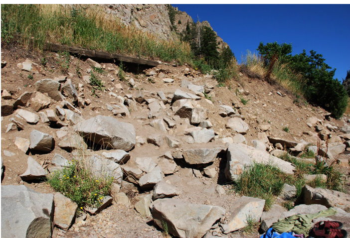
The hillside above the springs has eroded over time.
