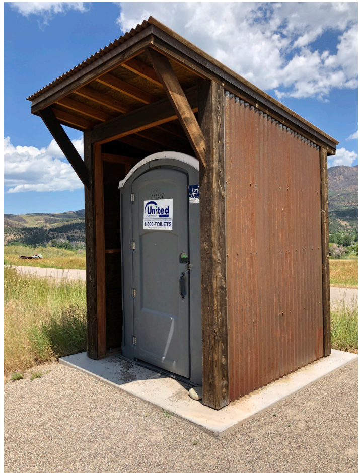
Example of the typical OST bathroom shelter installed at the Basalt High School Trailhead.
