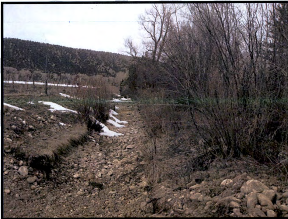
Photo 9. Table 1, Unit 8. Ditch size prior to piping is 8' wide x 2.5' deep. Head-gate dimension is 6' wide x 3' deep. This photo compares the old ditch size to the floodplain area and vegetation that was removed to install the irrigation pipe.
