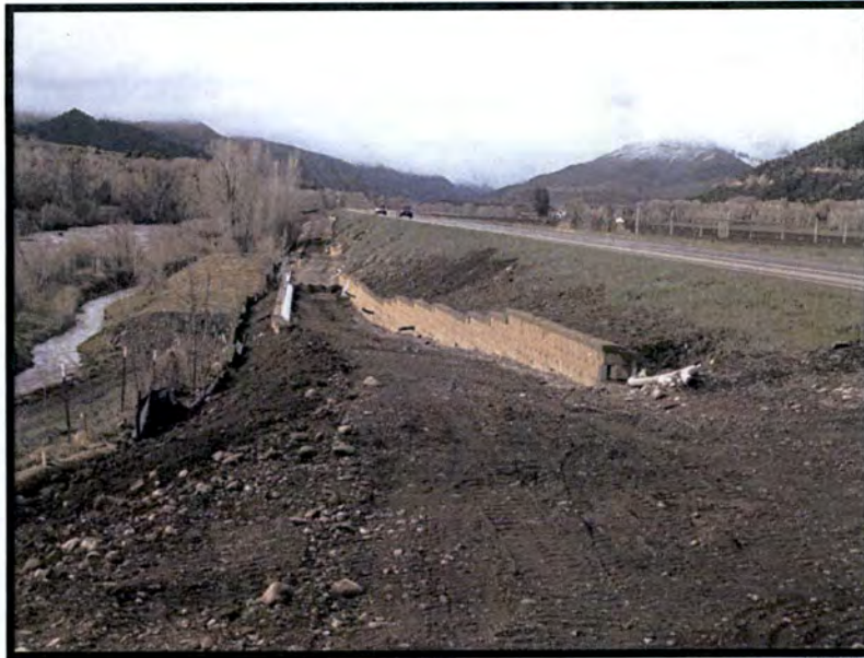
Photo 26. Table 3, Unit 6. This section of elevated trail is 932' long with a break in the center for 50', opposite the irrigation collector. It is not known if this section will also have a guard rail on the highway. Note distance between the pasture fence and the elevated rail vertical wall (discussed in Photo 25). Other barrier/obstacle impacts to wildlife have been previously discussed.
