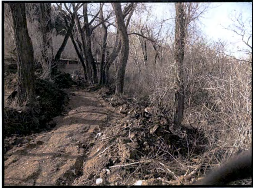
Photo 16. Table 1, Unit 10; Table 4, Units 1 and 2. Pipeline excavation at the north end of the wetland shown in photos 12, 13, 14, and 15. Trail prism is in the far upper left of the photograph and adjacent to the highway where the orange cone shows up in the photo. The 3 rd elevated trail section begins at the orange cone area. Note the larger cottonwood watered from ditch seepage before it was piped. Compare these cottonwoods with the smaller ones shown in Photo 17 that were not watered because the ditch went under highway. Large cottonwoods provide valuable wildlife habitat, particularly cavity nesters and raptors that use these trees for roosting and foraging. The elevated section of the trail is on the east side of the highway between the highway and the spindly cottonwood section as shown in Photo 17. No sediment fence.
