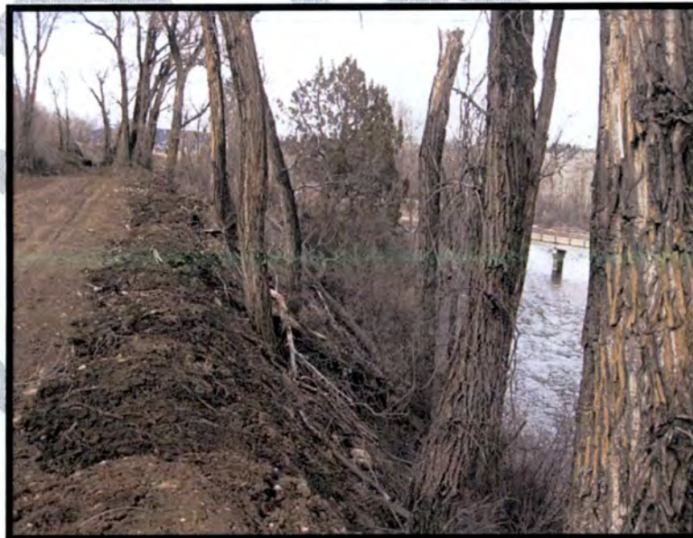
Photo 23. Table 1, Unit 15. Photo taken from same location as Photo 22 looking south to north. Thomas Creek Bridge is on the right side of the photo. Twenty foot wide vegetation removal to pipe an 8' ditch. Vegetation between new trail/pipeline and river will die back from dewatering thus reducing shade, mature cottonwoods, and wildlife trees for cavity nesters. Erosion into the river could potentially increase from vegetation reduction between the trail/ditch and the river. No sediment barrier was used in this section.
