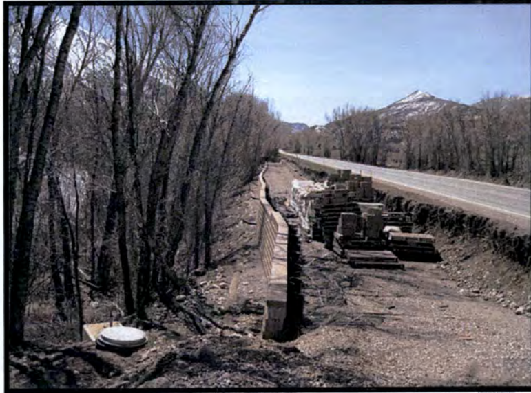
Photo 18. Table 1, Unit 11; Table 3, Unit 3. Looking south at elevated bike path. Old ditch now piped crosses back under highway. Note cleanout manhole. Pipeline continues north in front of new house and is piped to Thomas Creek Road. Prior to the trail the ditch was open just north of the house and before the house was built in 2008 the ditch used to run to Thomas Creek Road. Now it is piped for 475', 200' in front of the house and for 1,025' under the new trail prism for a total of 1,700'. Note elevation drop from highway to trail and imagine a guard rail on the highway and a 5' trail safety fence on the river side of the trail. This will be what wildlife will have to navigate around causing physiological stress. There will be more wildlife/traffic interactions because the confused wildlife will spend more time on the highway.
