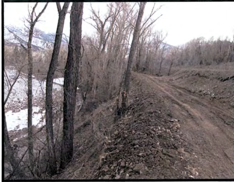
Photo 22. Table 1, Unit 15. Same prism as Photo 21 looking from north to south. In addition to piped length disused in previous photo this section is 519' for a total of 1,025' of piped ditch between the new house and Thomas Creek Road. Including all sections piped this totals 1025' (house north) plus 675' (house south to the wetland located in the northern end of the field north of Thompson Creek) for a total of approximately 1,700'. This will alter the remaining vegetation adjacent to the ditch/pipeline as discussed. In addition, the amount of vegetation removed in this section totals 6.075 sq ft (calculating for a 20' to 30' corridor for the pipeline/trail prism and reducing this by 10' to account for the ditch profile). Additional vegetation removal also occurred for pipe storage and staging with an additional 1/3 more of disturbed ground bringing the total to approximately 9,000 sq ft (0.2 acres) of disturbance in this short reach (under 1/4 mile). No sediment barrier was used in this section.
