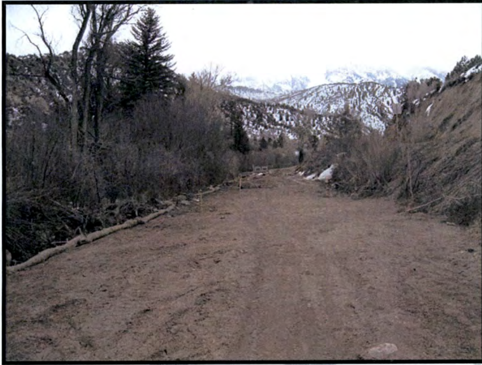
Photo 8. Table1, Between Unit 7 and 8. Looking south towards new diversion dam. At the north and south ends of this activity the riparian and other vegetation was removed for more than 50' in width. Pipe exits to the north of the photo, not seen in photo.
