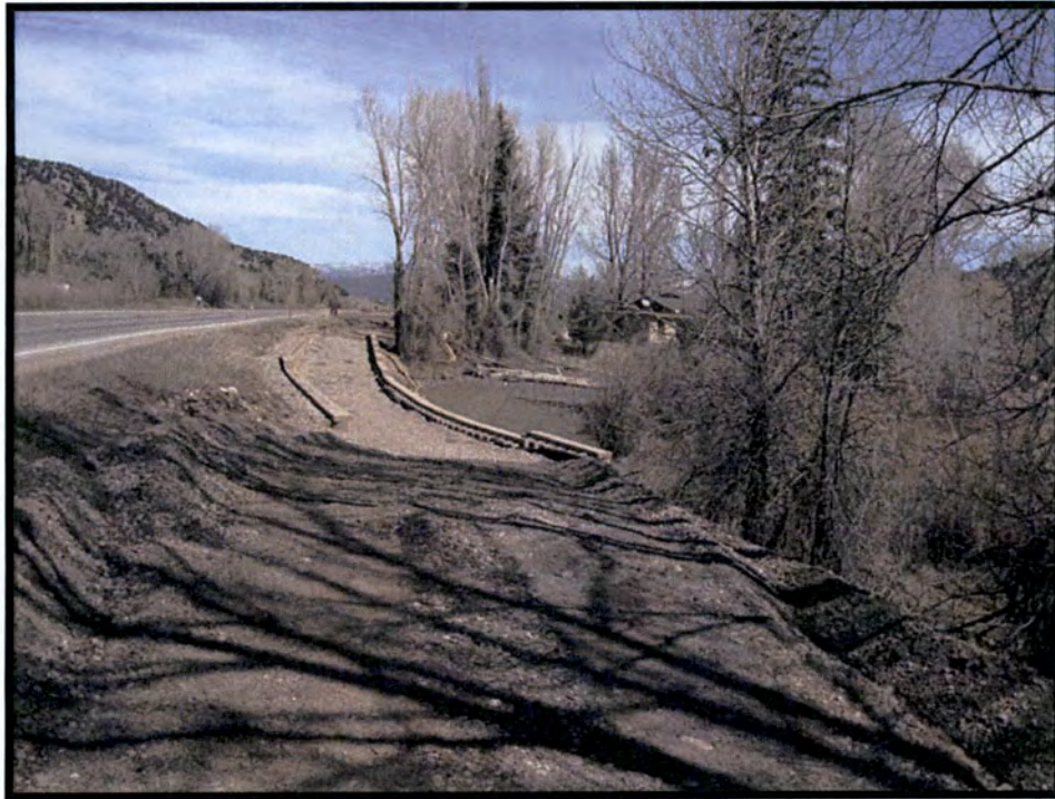
Photo 10. Table 3, Unit 2. (EES wetland report Figure 13). Elevated trail section along the wetland and pond. Fill in bottom right of photo and along pond edge. With the new trail adjacent to the wetland and pond, wildlife and wading birds will be disturbed by human activity limiting their foraging ability.
